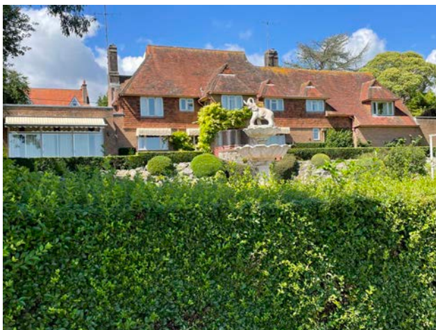
Rear elevation overlooking Clays Field
